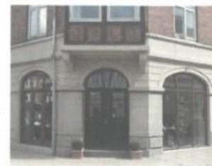
Rehabilitering, Restaurant Luce, Hviding
